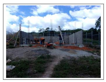
**Above:** The kindergarten with one wall built. **Below:** The kindergarten with three walls built. The windows will be in the front and back; the doors will be in the front. This week they are pouring the columns and the beam to go on top of the wall.
