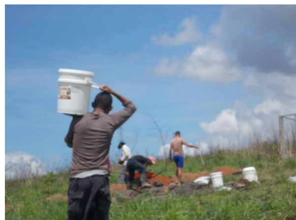
Top: The kindergarteners receive bags of hygiene kits from Christ Child Society. It's their first time to have their own soap, shampoo, washcloth, comb, toothbrush and toothpaste. Below: Carrying water to the construction site. The town water system can supply very little water to the homes.
